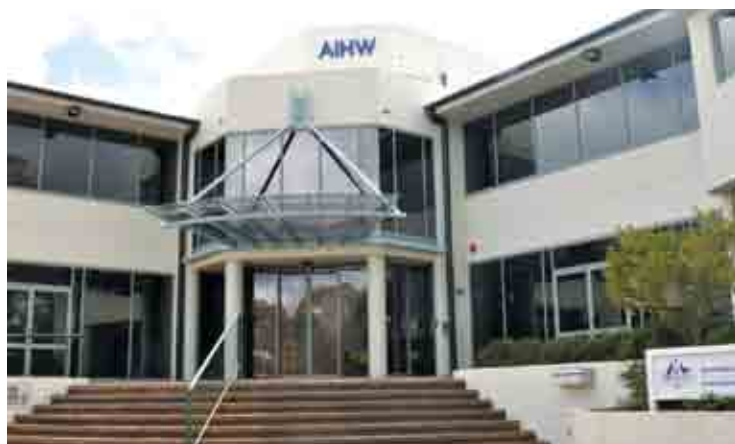
The AIHW main building at 26 Thynne Street, Fern Hill Park, Bruce.
