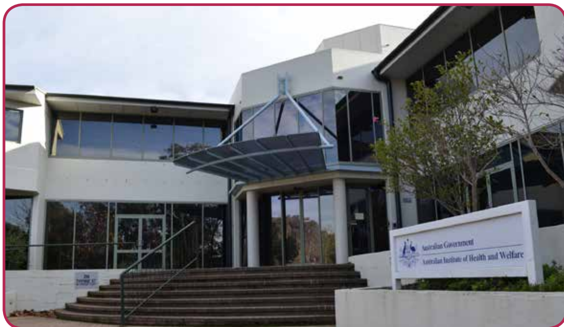
The 'old building': the main AIHW building at 26 Thynne Street, Bruce.
