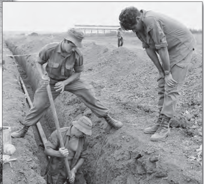
Soldiers install a water system for a village in Phuoc Tuy Province. [COM/69/0005/VN]
